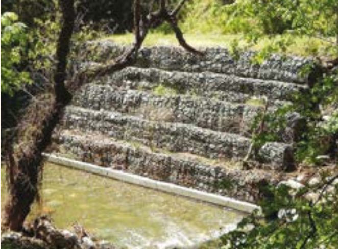
Gabion teras duvar
